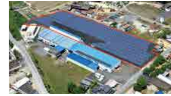
Solar power generation equipment at Inoue Jikuuke Kogyo Co., Ltd.
