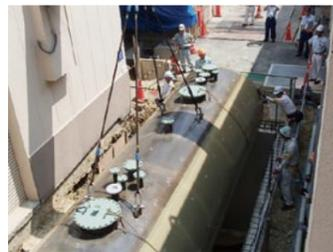
Photo 1: Switching to a double-hull tank
