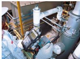
Measuring exhaust gas and optimizing firing conditions
