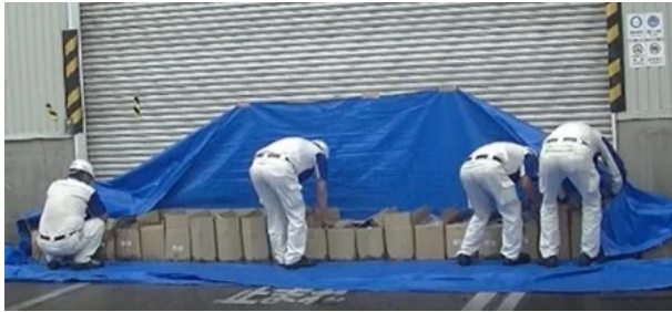
Regular training on installing anti-flood plates
