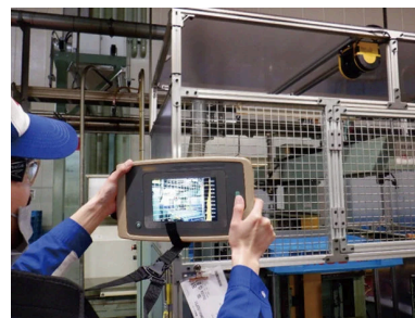
Air leak detection at the Ishibe Plant
