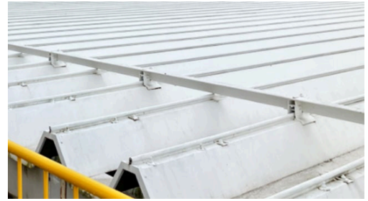
Thermal insulation coating on the roof of the Fukushima Plant
