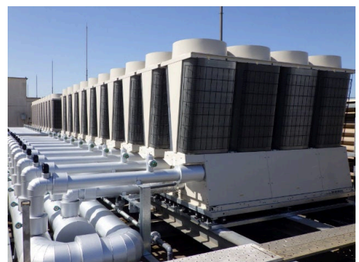
Air-cooled chillers installed at the Saitama Plant
