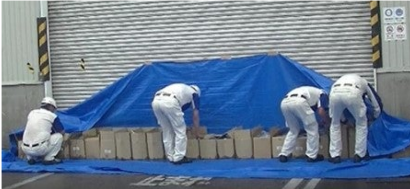
Regular training on installing anti-flood plates
